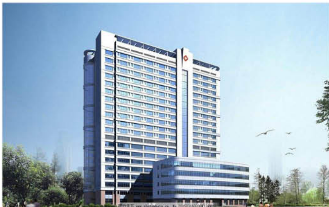
The Hospitals Wall cladding
